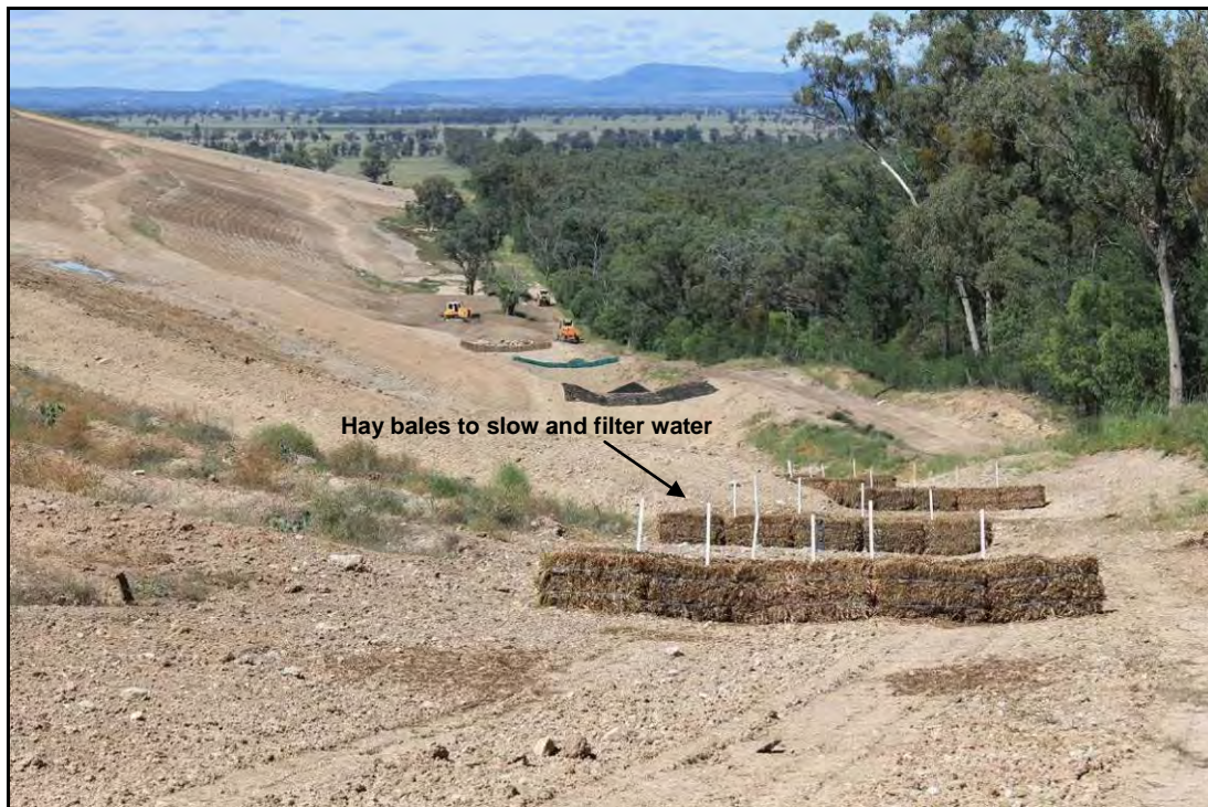
Plate 3 – Hay Bales Used to Control Erosion and Sedimentation, March 2012
